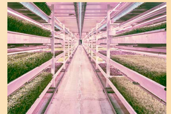
Lighting for plants in vertical farming is placed underneath the floorboard of the shelf above. Image of Underground Growing Farm, London - Courtesy Valoya - www.valoya.com
